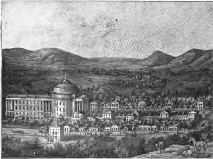
THE UNIVERSITY OF VIRGINIA As designed by Thomas Jefferson
